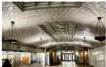
Hartford City Hall Renovation Hartford, CT
