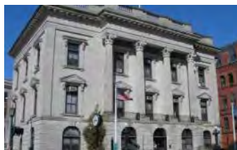
City Hall Vault Demo & Alteration New London, CT
