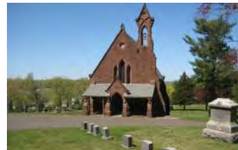
Indian Hill Cemetary Chapel Restoration* Middletown, CT
