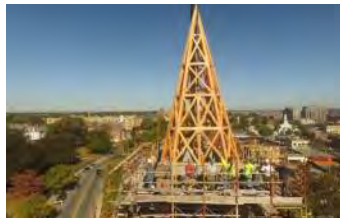
Grace Episcopal Church Spire Reconstruction* New Bedford, MA
