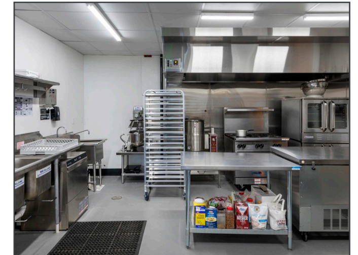
USDA certified commercial kitchen on ground floor
