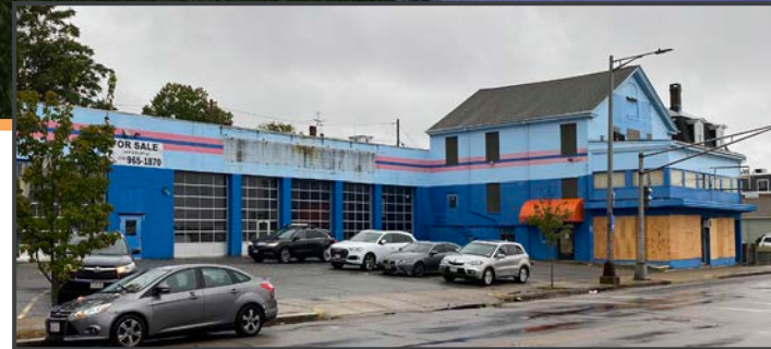
Existing exterior conditions
