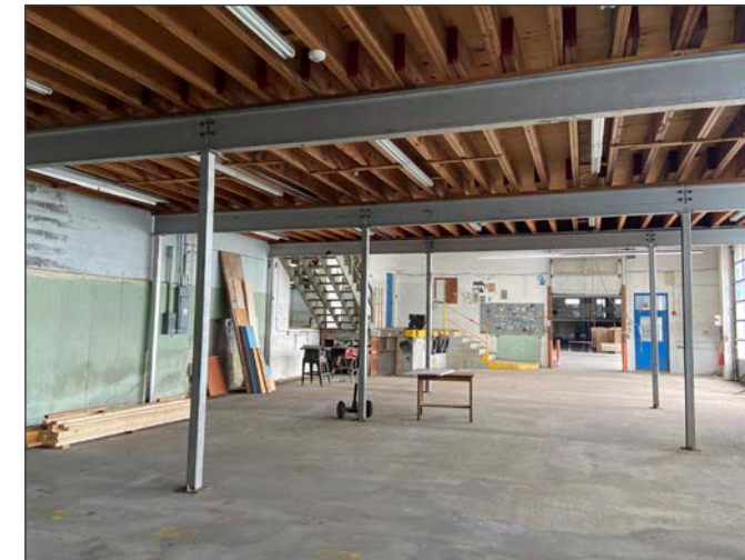
Existing interior conditions
