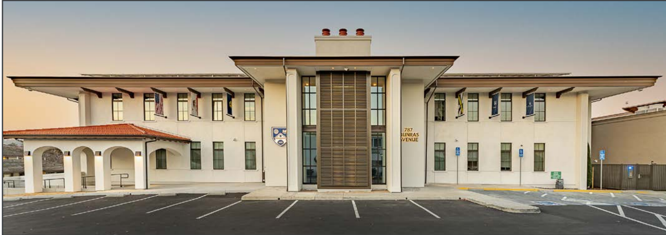
View of renovated exterior
