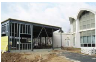
St. Mary Mother of Redeemer Church Parish Hall Addition Groton, CT
