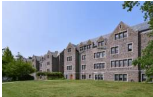
Quad Dormitories Assessment & Repair Connecticut College New London, CT
