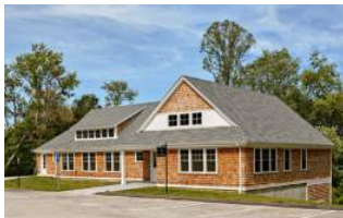
Hillel House Connecticut College New London, CT
